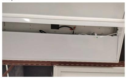
7) Put all showed wires back outside to inside of fixture to hide them(Not let them to effect the main part installed). And then rotate central light engine part to horizontal place and then push it a little to make it secured with 2 end bracket parts
