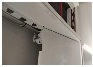
3) Install another long side part to another side similarly where is sitting EM driver, to hide the EM driver but take out the wires from EM driver and show, including two plug wires and one indicated light wire
